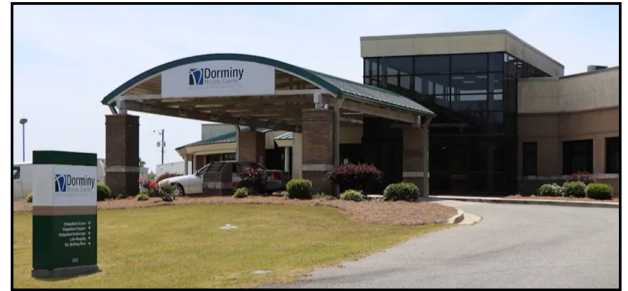
Dorminy Medical Center's Rehab Facility
